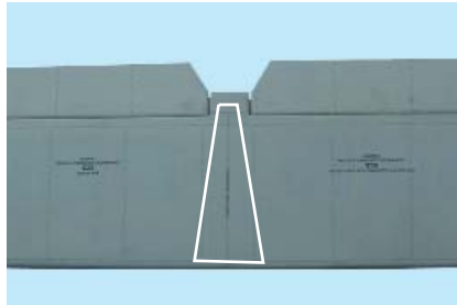
8.1 Marked lines on horizontal stab
