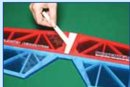
8A. Apply plenty of epoxy
